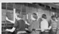
Operator Switching Stations
